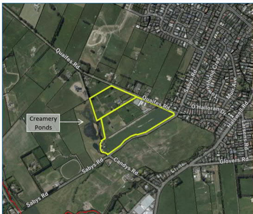
Aerial image of site from Canterbury Maps, aerial taken November 2018
